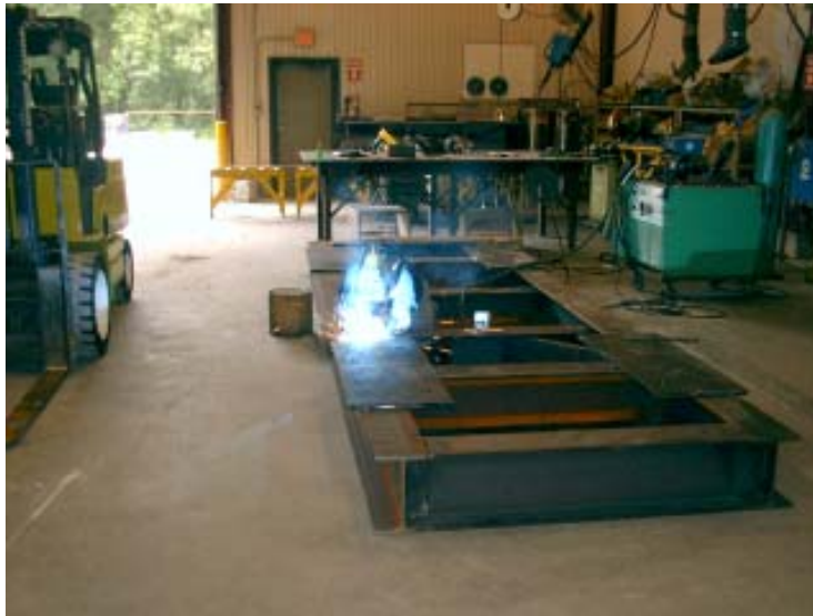
Brad Arkland is pictured welding on the motor base structure for the Martin Marietta plant in Fort Dodge, Iowa.
