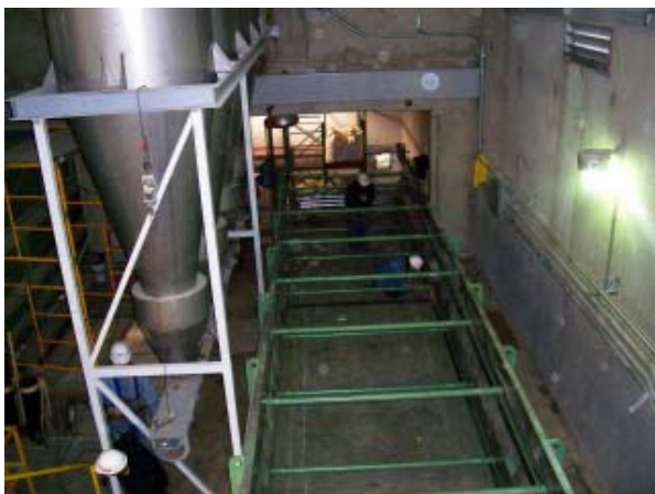
T&S crews shown above are assembling the CPM 85 TPH horizontal cooler.
