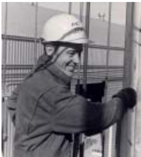
1970 - Art working on the Ceres Land Company slip in Sterling, Colorado.
